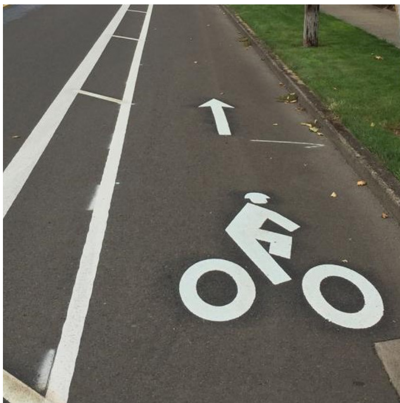
Figure 5.4: Buffered Bicycle Lane
