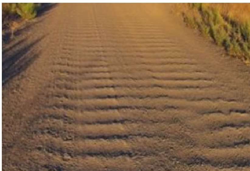
Figure 3.16: Washboarding (source: Landlock Paving)
