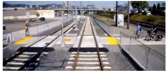
Figure 2.22: Sample At-Grade Rail Crossing Treatments (source: Trimet)
