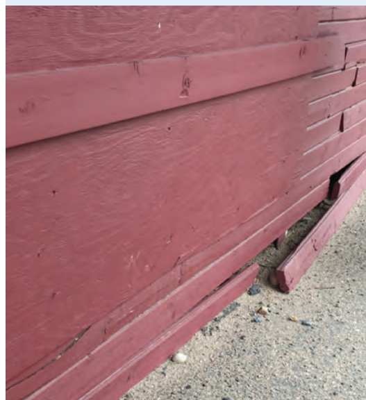
THE TONGUE AND GROOVE WOOD SIDING IS DETERIORATING
