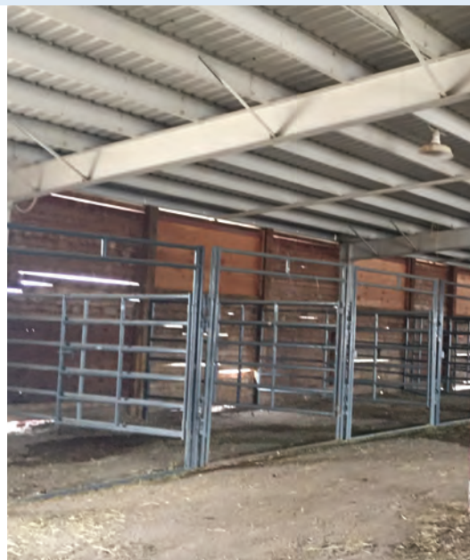
THE TONGUE AND GROOVE WOOD SIDING IS DETERIORATING
