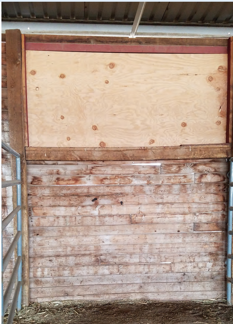
EXPOSED PLYWOOD PANELS TO KEEP OUT WINTER CONDITIONS, REMOVED IN SUMMER FOR VENTILATION
