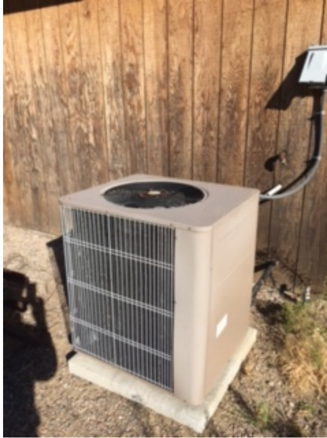
Air conditioning unit with potentially containing Freon
