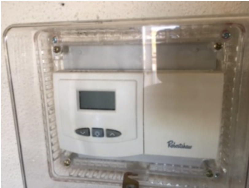
Typical wall-mounted thermostat potentially containing mercury
