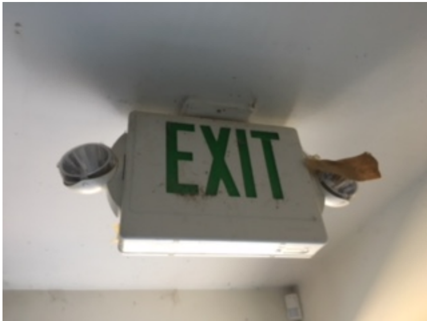
Typical emergency exit sign with potential radioactive isotope
