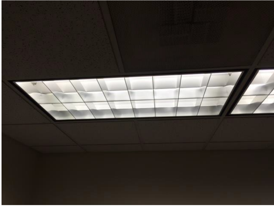
Typical lighting with potential Hg lightbulbs and PCB/DEHP ballasts
