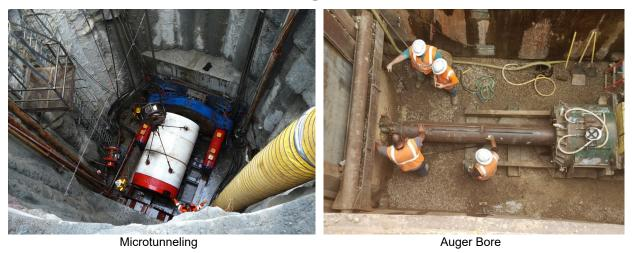
Figure 7-1: Example Trenchless Construction Method
