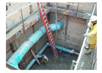
Figure 10-10: Example of Tunneling Pit (for trenchless construction)
