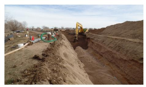
Figure 10-9: Examples of Open-Cut Construction Methods
