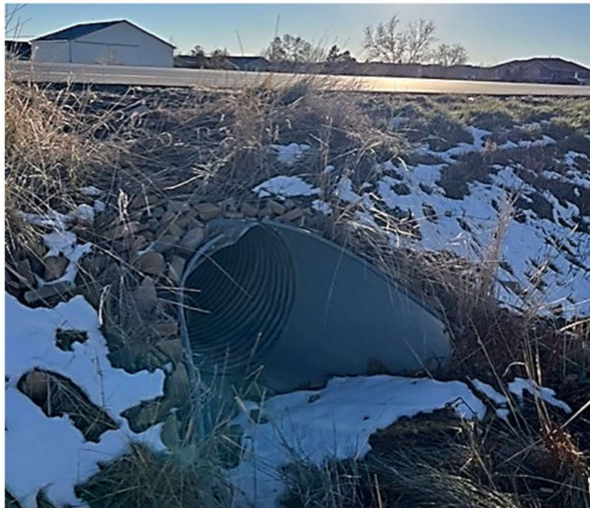
Photo 5 – E.160 th Ave. 36-Inch Dia. CMP Culvert Photo Perspective: Looking South; A.Cvar, 2024-12-05
