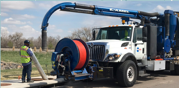
Example of urban storm sewer cleaning of inlet at Gilpin St. and SH 224 by Pro-Pipe Contractor in 2018 using a vacuum jet-truck.
