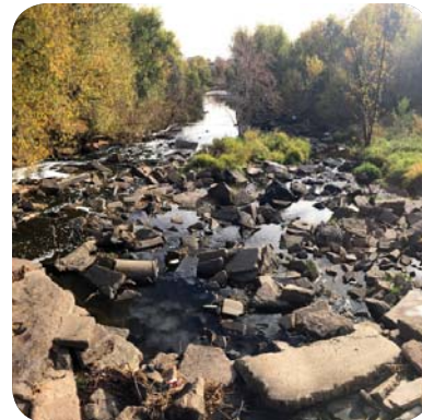
Riprap throughout streambed limits access for recreation or maintenance
