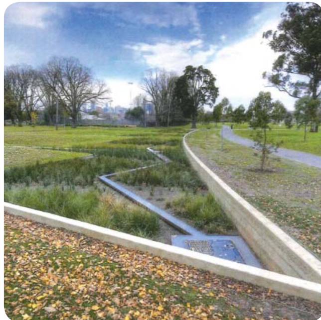
A well-designed stormwater outfall - pulled away from frequent flood zones and easily accessible for maintenance teams
