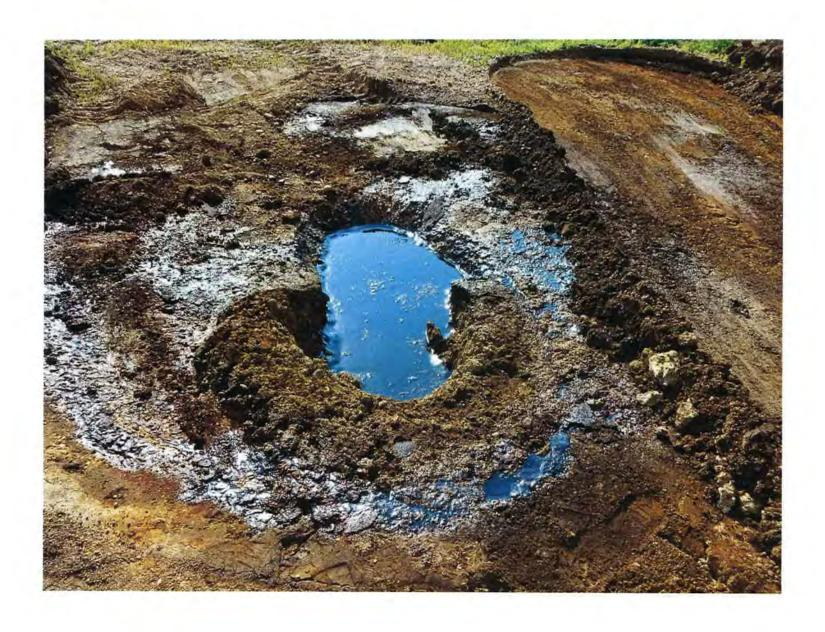
3 Phase flow line from wellhead to separator was located and found to include pneumatic controls gas line returning from the separator back to the wellhead to operate pneumatic valves, both removed.
