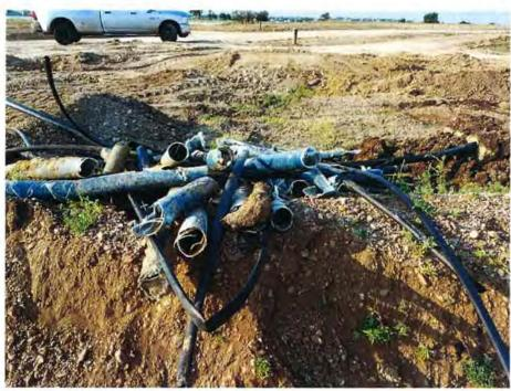
The bulk of the 3 phase flowline was 3" fiberglass with a black plastic pipe presumed to be pneumatic controls.
