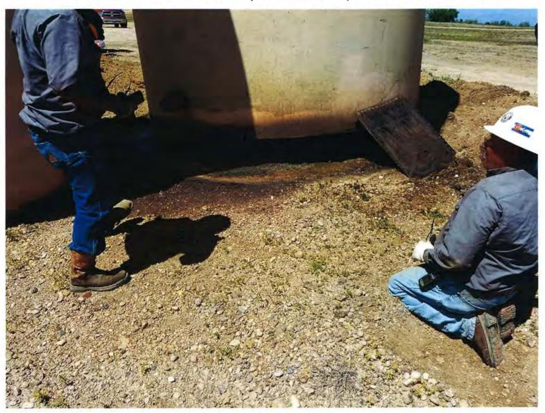
Tank was laid on its side to get it out of the sump depression in the ground under the tank. That depression had several inches of green/black (Sussex) crude oil standing in it. Contractor sucked this oil up with a vac truck.
