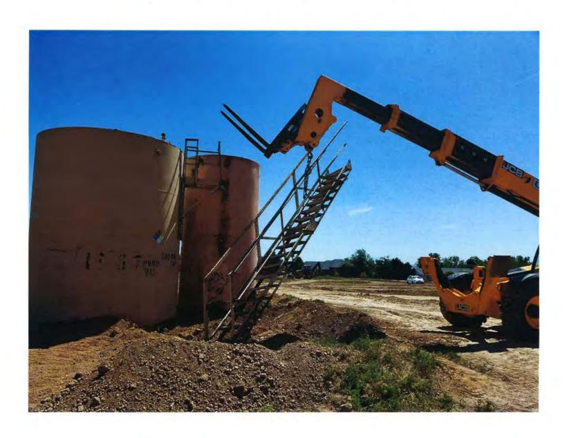
The contractor attempted to slide the tank away from the battery site to avoid cutting the tank apart near the contaminated soil.
