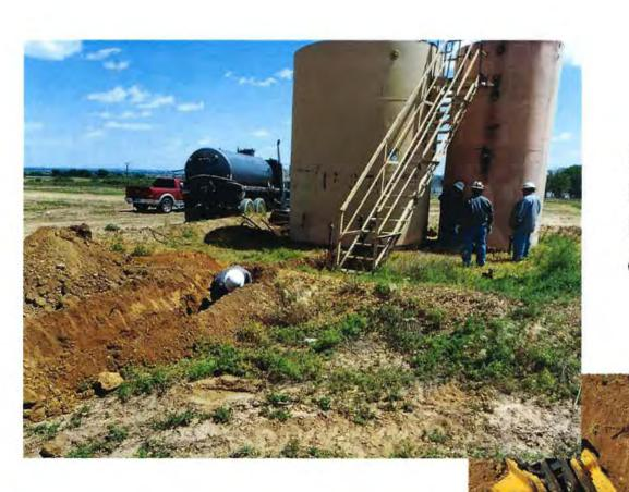
Removing on-site flowlines between separator and tank battery. Soils do not appear contaminated here.
