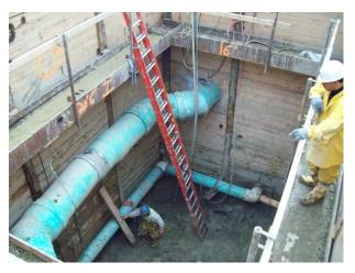
Figure 10-10: Example of Tunneling Pit (for trenchless construction)
