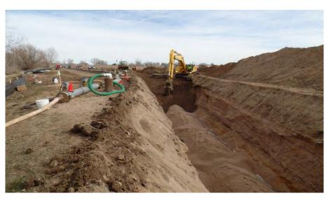
Figure 10-9: Examples of Open-Cut Construction Methods
