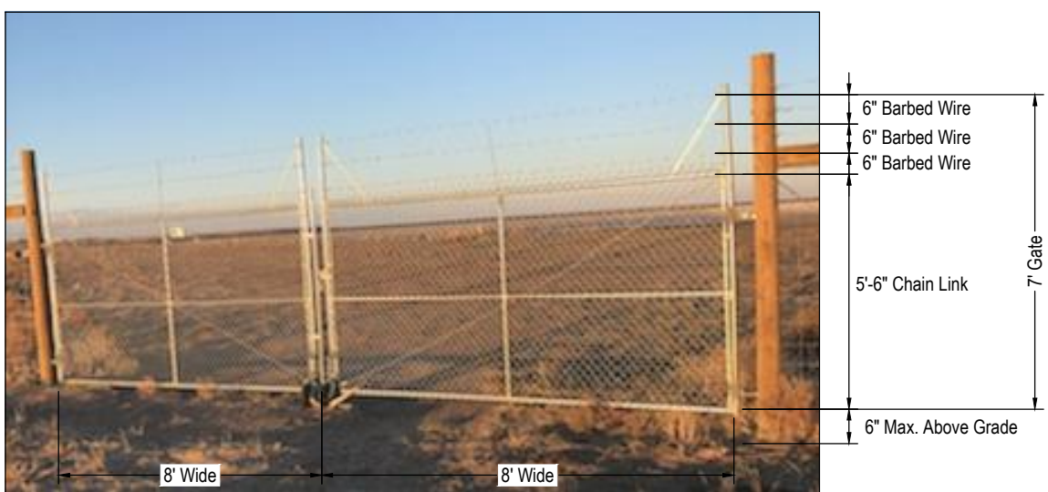
CHAIN LINK GATE DETAIL
