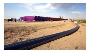
Surface frack water pipeline in Weld County
